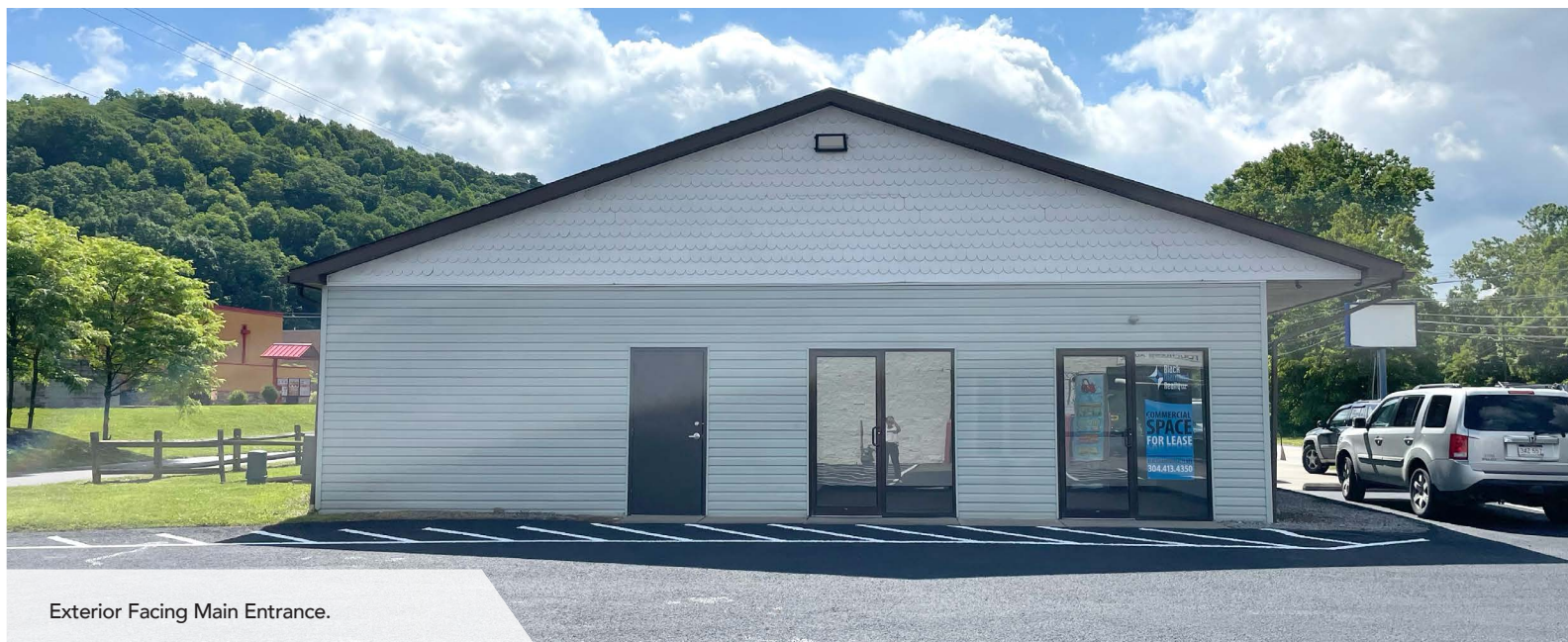
Exterior View Facing Greenbag Road.
