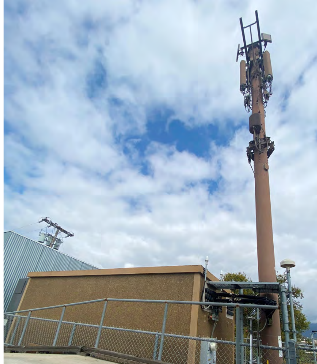
Cell site & loading ramp shown above. There is currently an offer to buy out the cell tower lease for $625,000, which a new owner could potentially use to their advantage.
