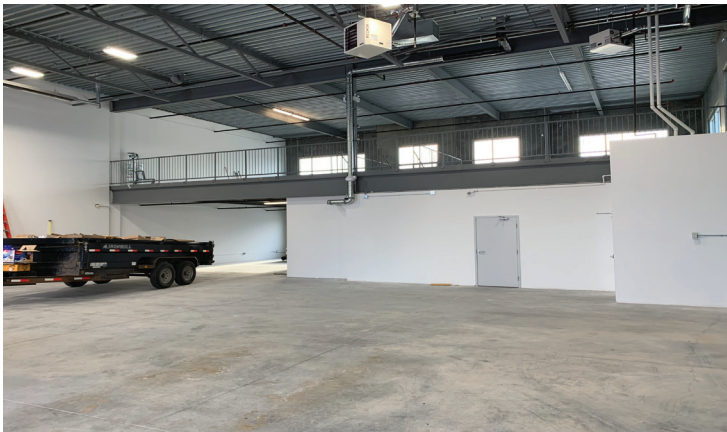
Bay with mezzanine
