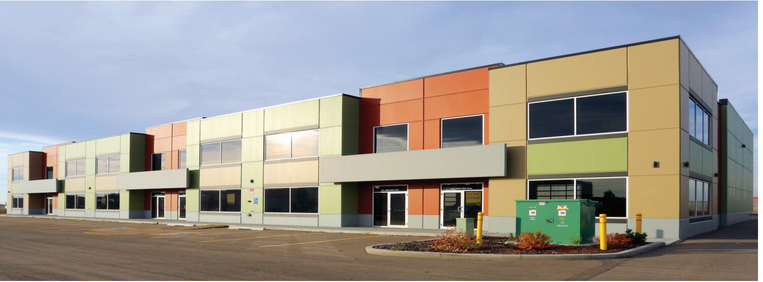
Overview of property
