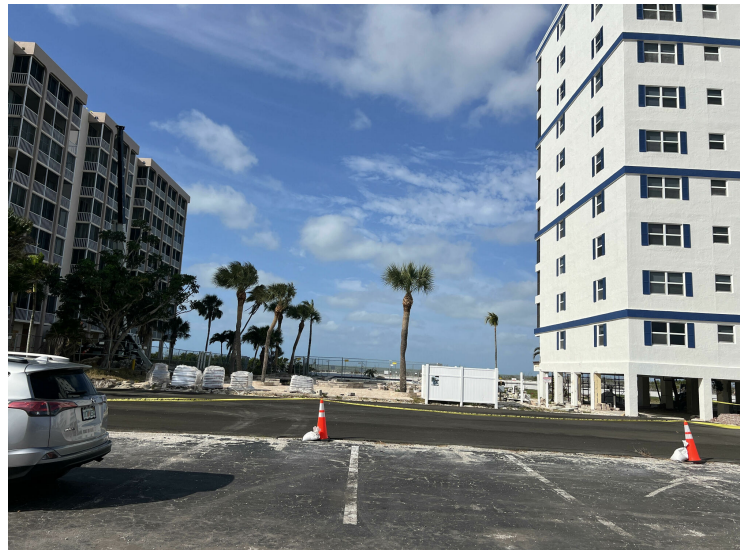
View from behind the building looking out to the beach.
