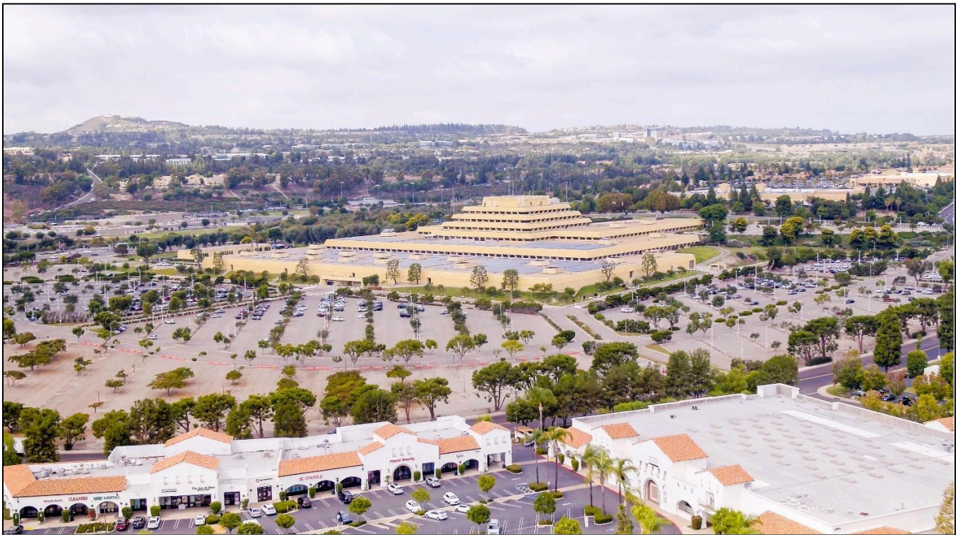
Aerial View to the Northwest
