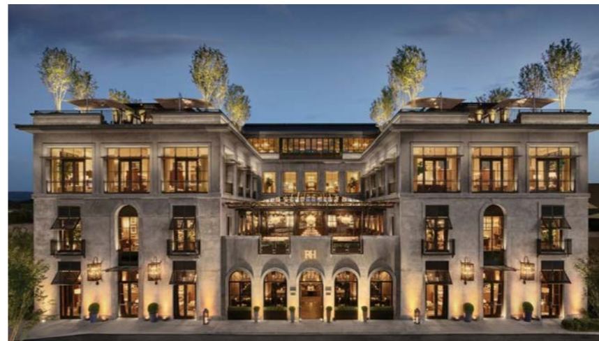
Restoration Hardware - Green Hills
