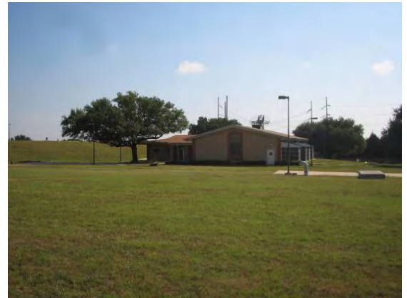
Dallas water utilities sump area located along Houston School Road should be preserved as green space.
