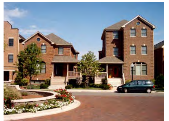
Moderate to high density townhouses and apartments should be located within walking distance of the proposed DART station. Source: Bridgeport Village, Chicago, IL
