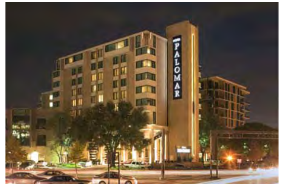
Higher density hotels and office complexes should be located within the Business Center development block.
