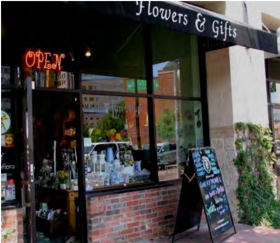
Create attractive and inviting street facing shop fronts as seen on Allen Street.
