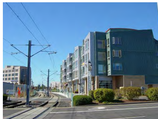
Transit station areas provide ideal location for higher density mixed-use development. Source: Beaverton, OH - Dan Tasman
