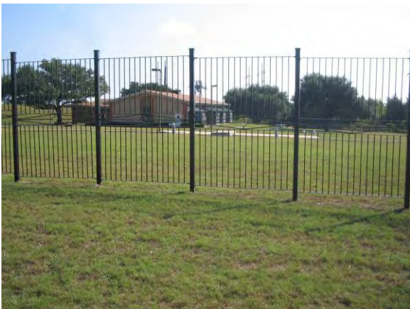
DWU sump facility as seen from Houston School Road
