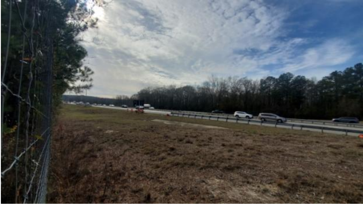
View of Interstate 75
