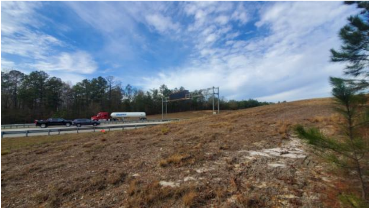
View of Interstate 75
