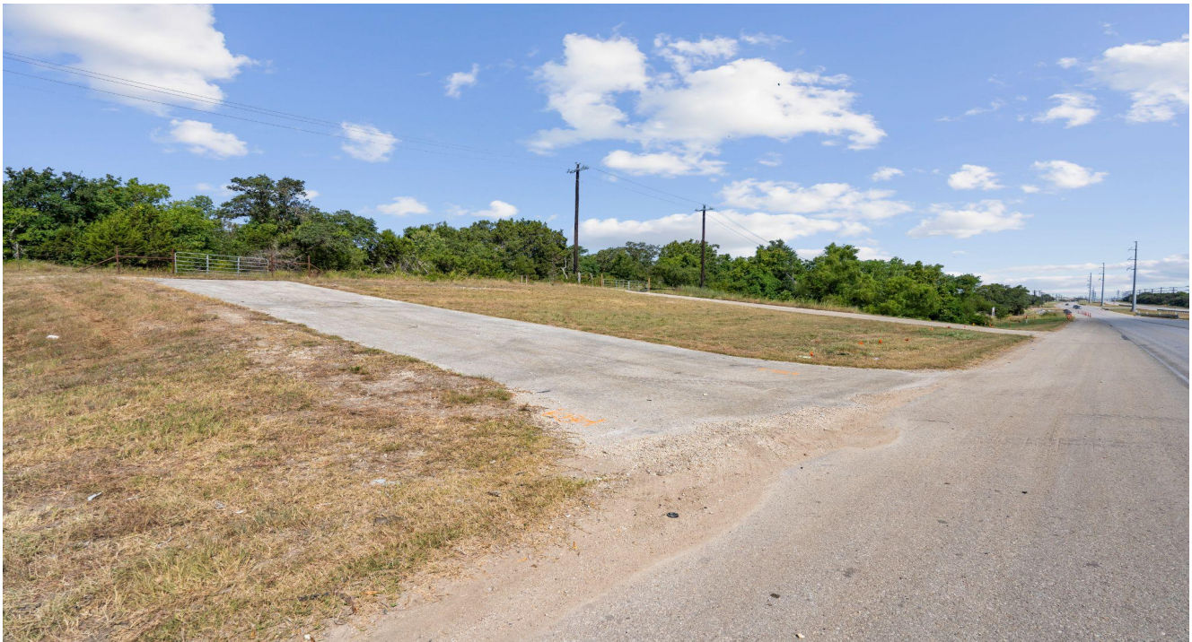
Lot 6 Access Road
