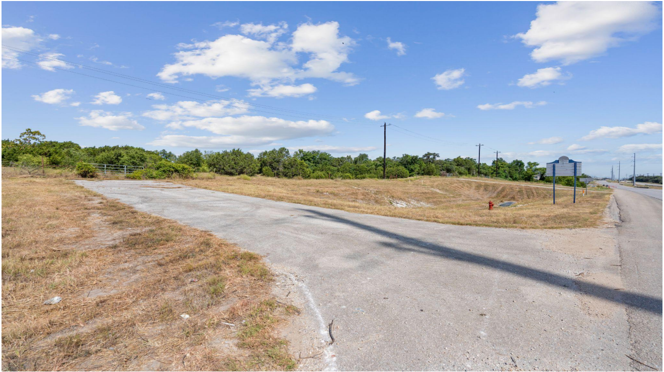
Lot 5 Access Road
