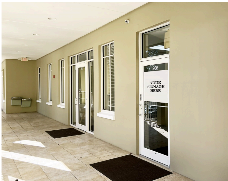
2nd floor Landing
