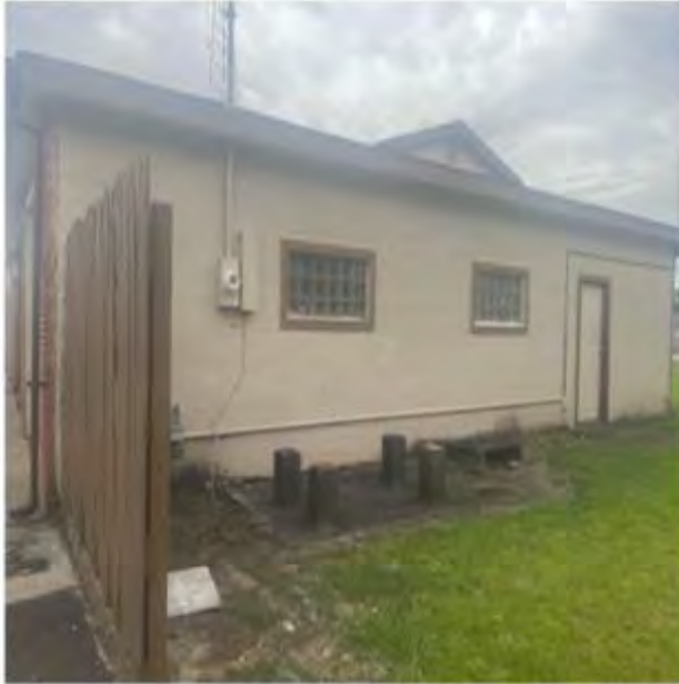
North side of the building
