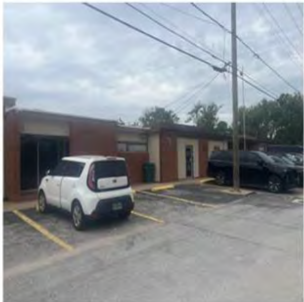
East side of the building
