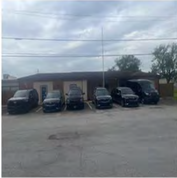
East side of the building
