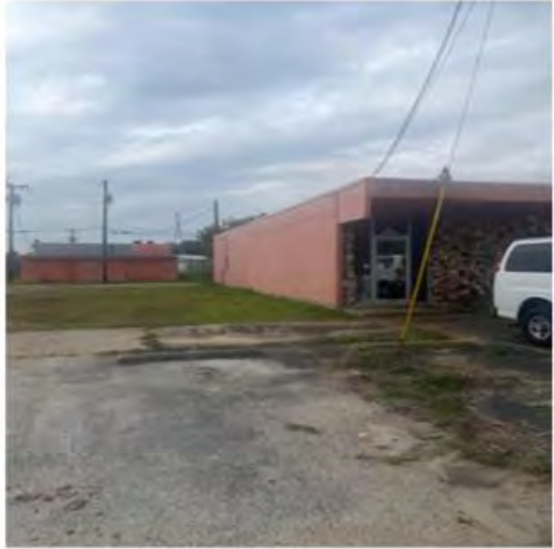
South side of the building
