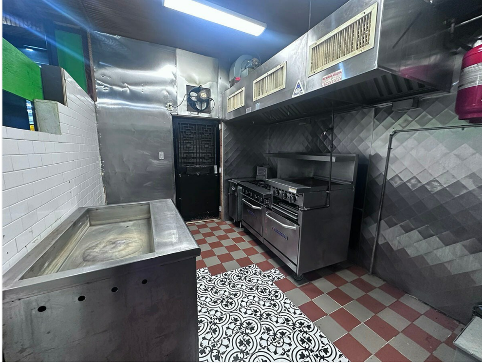
basement prep area
