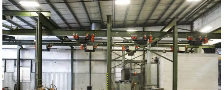
Trolley Room - secondary paint line will be removed
