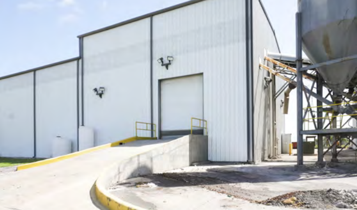
Loading ramp leading to Concrete Batch Hopper
