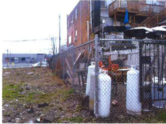
South Side of Site & Neighboring Property to the South
