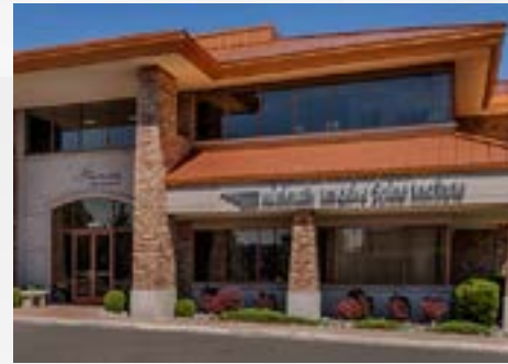
9990 Double R Blvd., Reno 20,549 SF Class A Commercial Office and Medical Building
