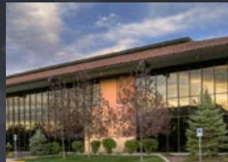
5370 Kietzke Lane, Reno 55,559 SF Class A Office
