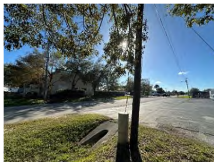
View From SE Corner of Subject Property
