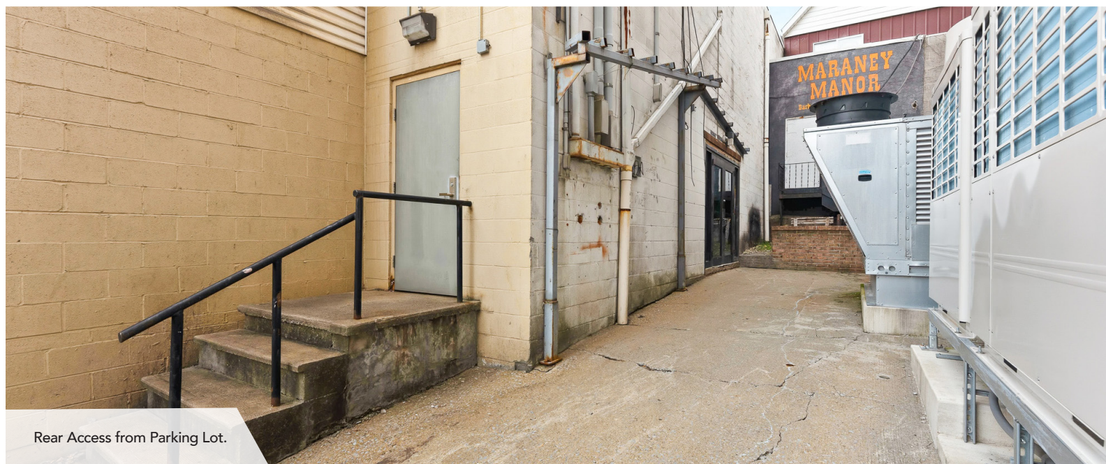
Rear Access from Parking Lot.
