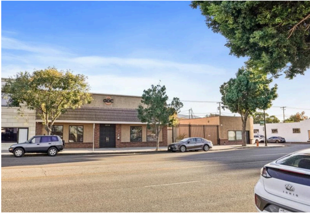
Front of Property
