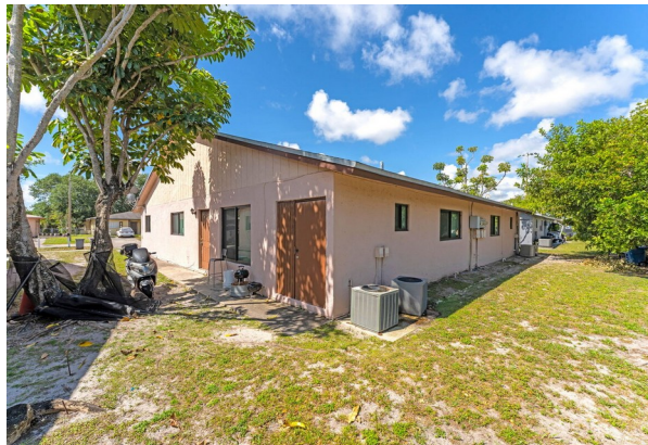
Rear Elevation & HVAC
