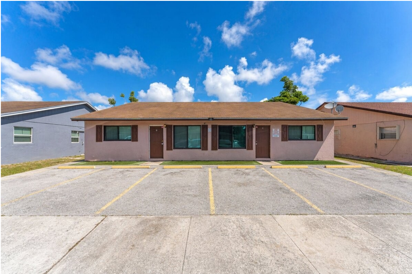
Front Elevation — 1481 NW 22nd Street, Fort Lauderdale, FL
