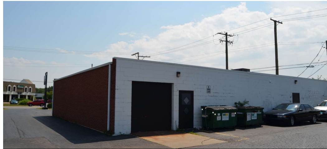
Overhead Door in Rear
