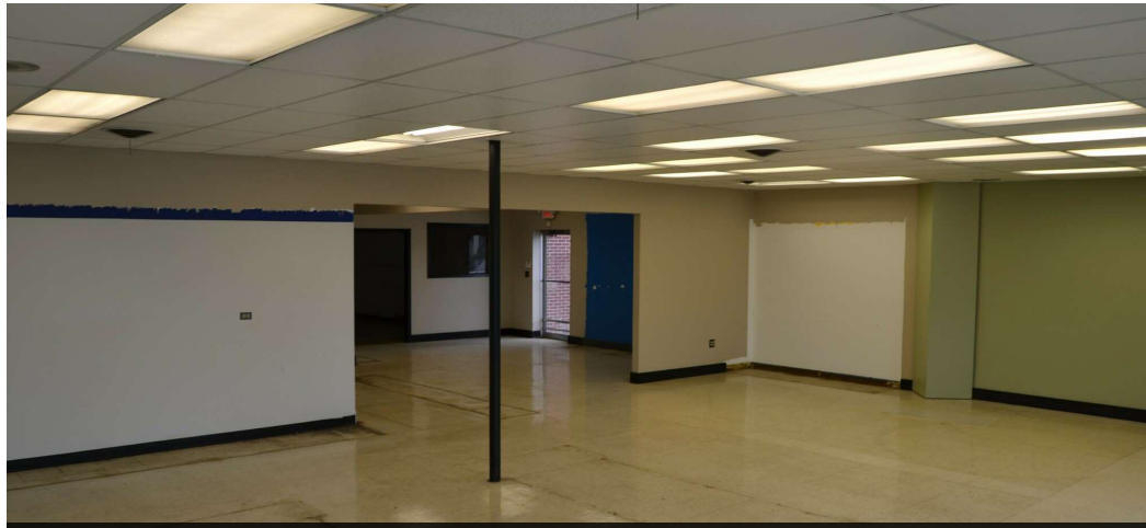
Lighting Grid with Acoustic Tile Ceiling In Place
