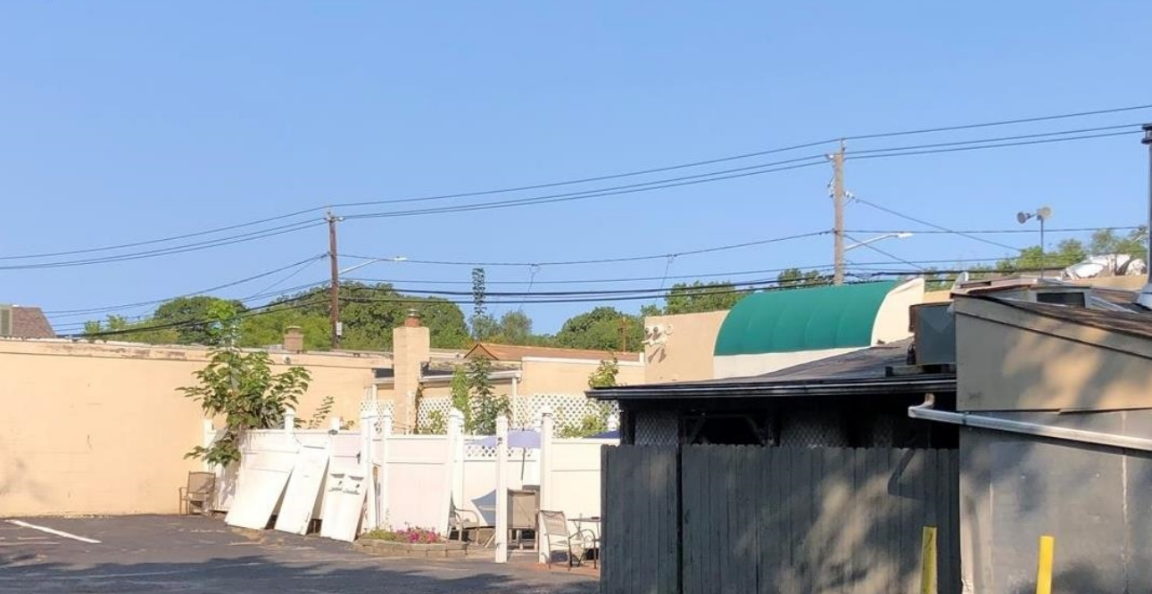
Back of Building
