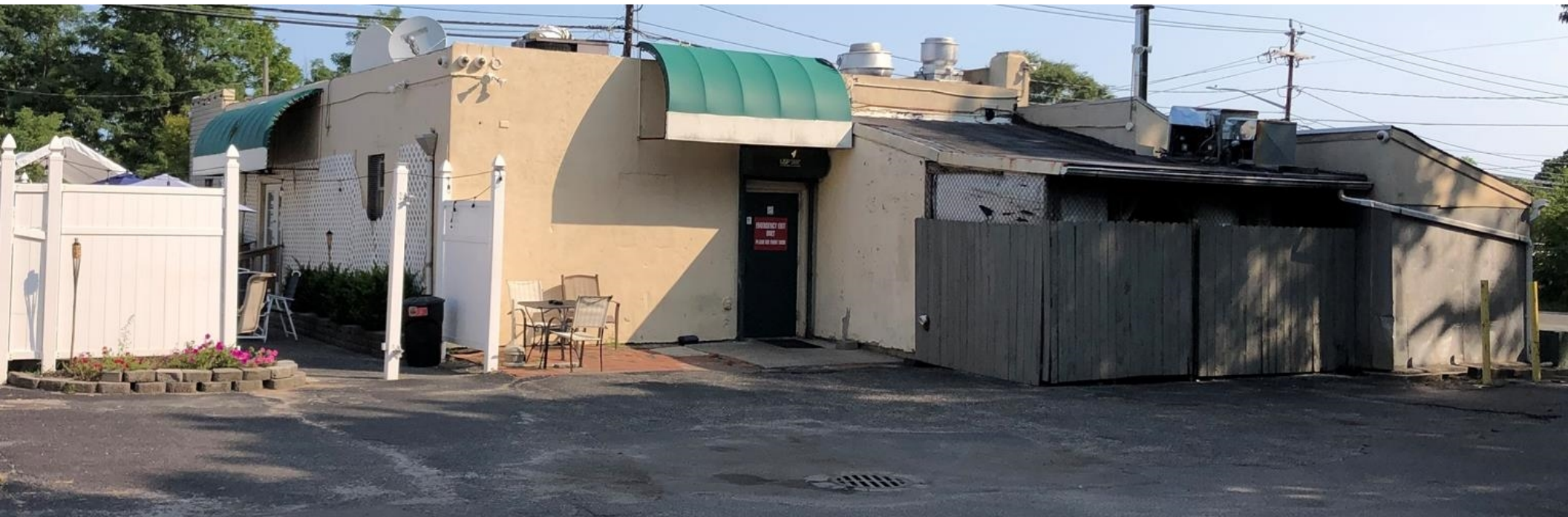
Back of Building
