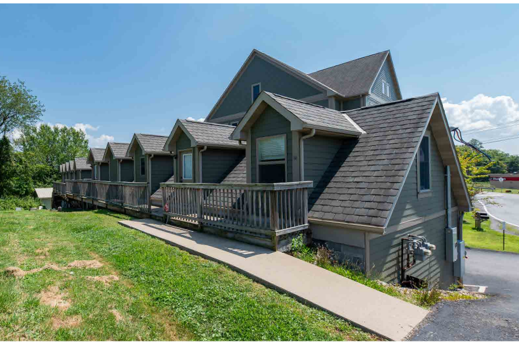
Access to Upper Levels of 8 and 10 Canyon Road.
