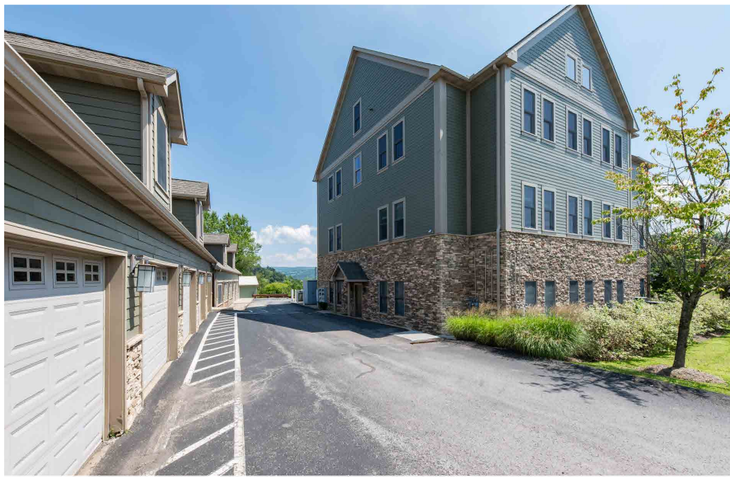
Lower Level View of 8 and 10 Canyon Road.
