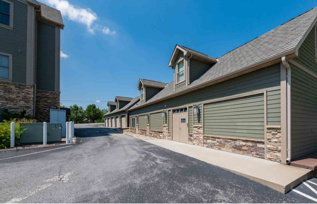
Lower Level View of 8 and 10 Canyon Road.
