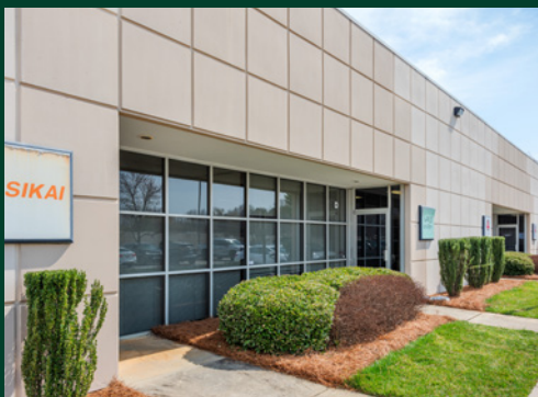
PRECAST CONCRETE AND GLASS FACADE
