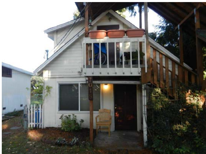
View of duplex exterior (Units 1 & 2)
