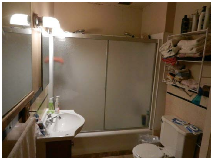
View of bathroom in Unit 4
