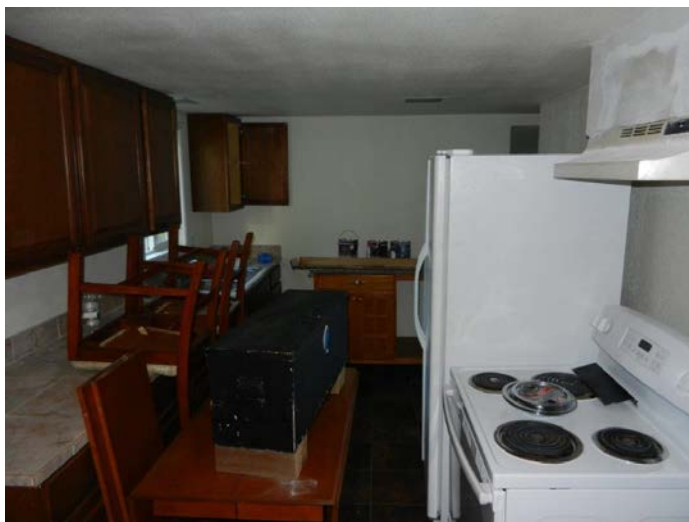
View of kitchen in Unit 1
