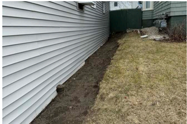
South wall prior to installed stone drip edge
