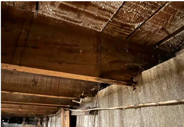
Existing joist seat at basement wall
