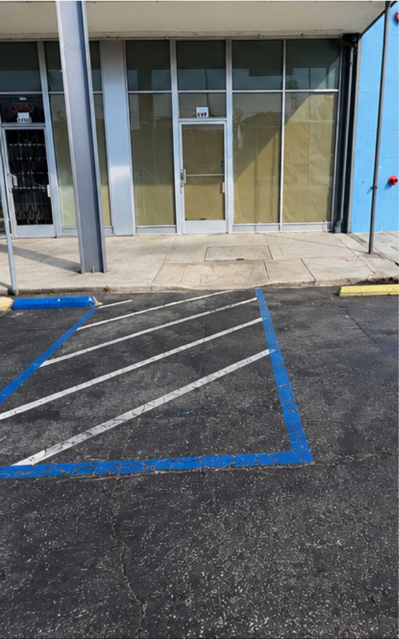
Unit C1 Main Entrance
