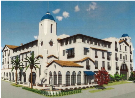
Address 800 Mission Avenue at Lincoln Ave Status Under Construction
