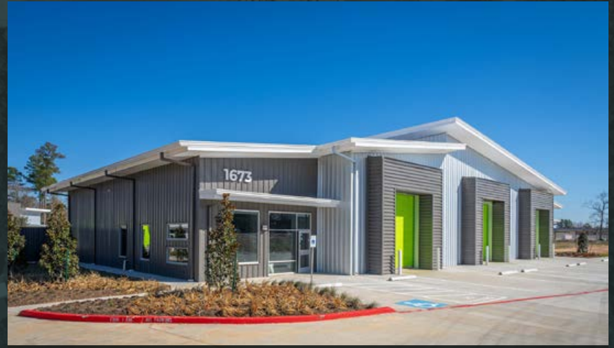
Modern Storefront Design with Prominent Tenant Visibility
