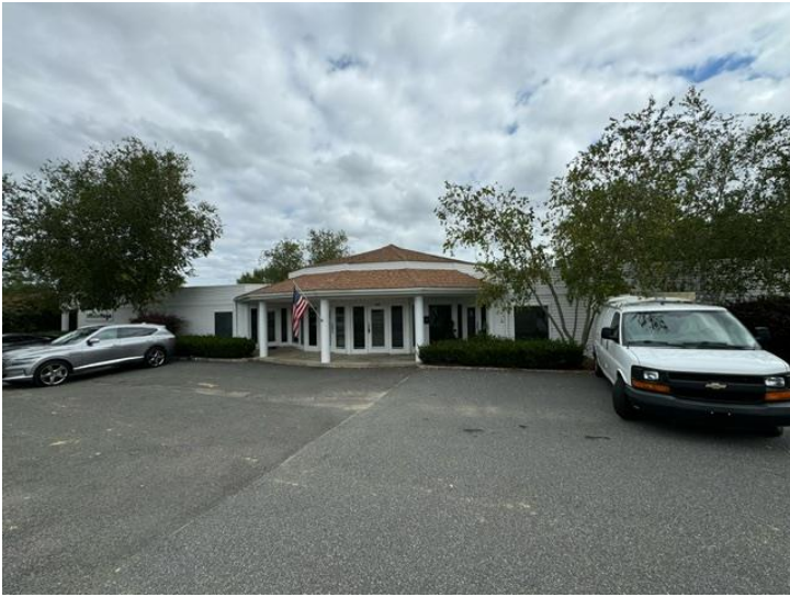
Main entrance of building
