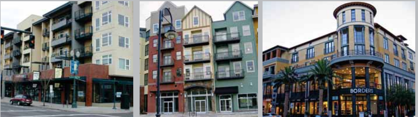
Example: Three or four stories of residential units (condos or apartments) above ground floor retail (cafes, coffee shops, boutiques).
