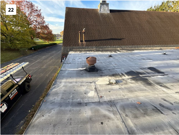
Project: Inspections (East Ave) Front Line Date: Nov 4, 2025, 8:15 AM Creator: Justin Moser
