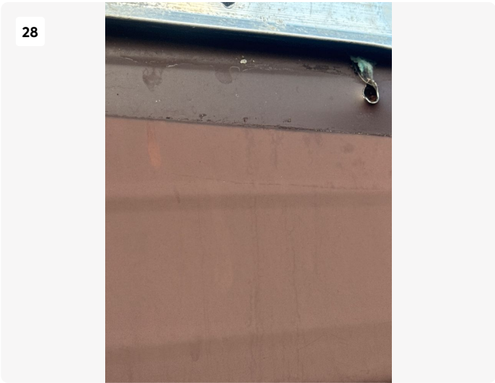
Project: Inspections (East Ave) Front Line Date: Nov 4, 2025, 8:18 AM Creator: Justin Moser
