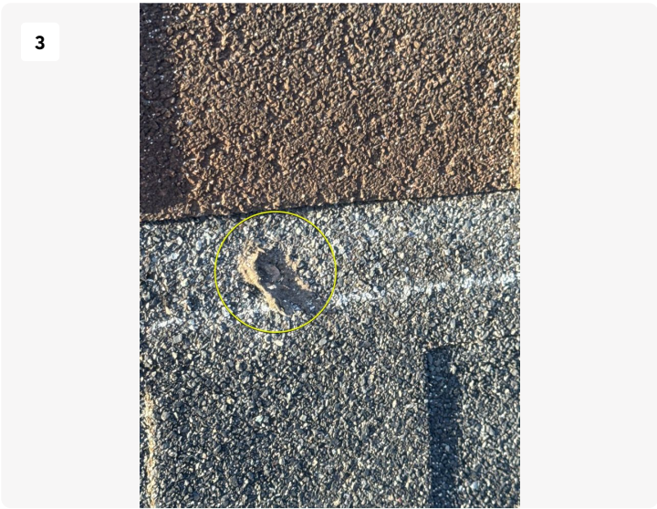
Project: Inspections (East Ave) Front Line Date: Nov 4, 2025, 8:11 AM Creator: Justin Moser
