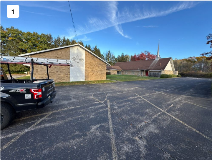
Project: Inspections (East Ave) Front Line Date: Nov 4, 2025, 8:20 AM Creator: Justin Moser
