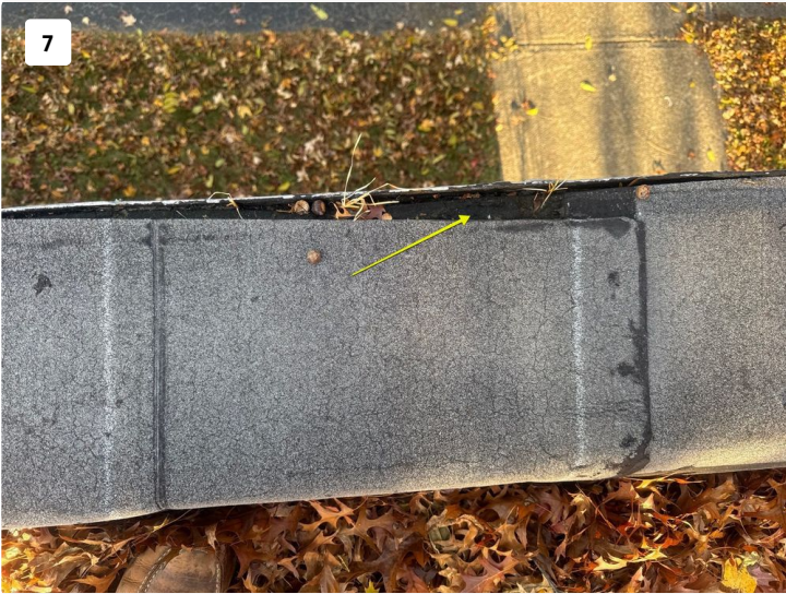
Project: Inspections (East Ave) Front Line Date: Nov 4, 2025, 8:12 AM Creator: Justin Moser
