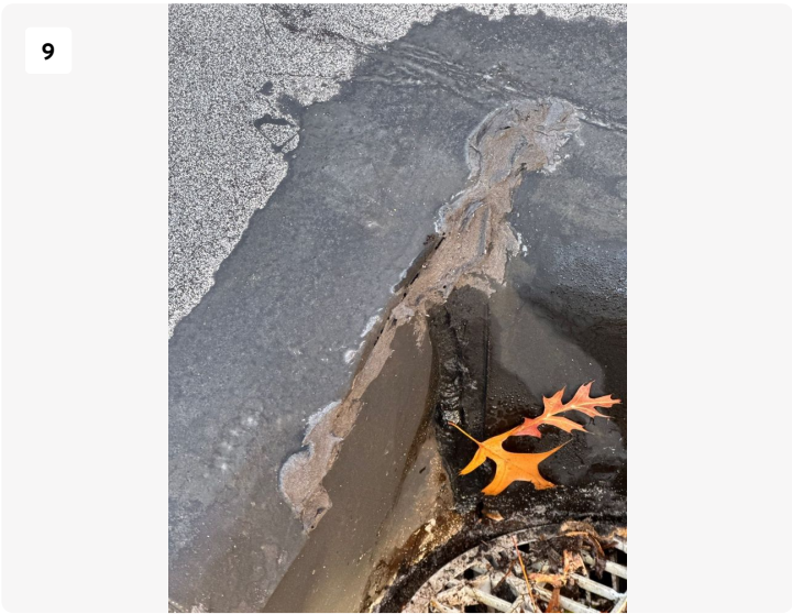
Project: Inspections (East Ave) Front Line Date: Nov 4, 2025, 8:13 AM Creator: Justin Moser
