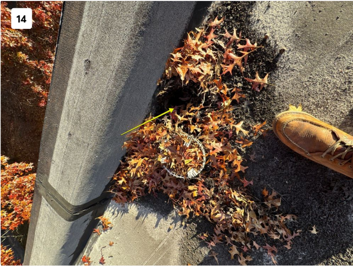
Project: Inspections (East Ave) Front Line Date: Nov 4, 2025, 8:14 AM Creator: Justin Moser
