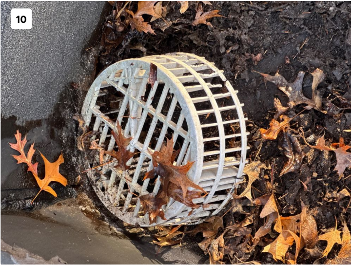
Project: Inspections (East Ave) Front Line Date: Nov 4, 2025, 8:13 AM Creator: Justin Moser
