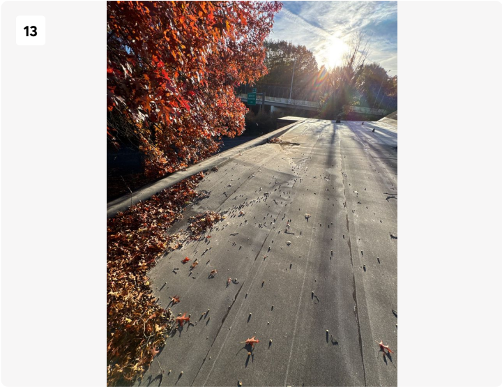
Project: Inspections (East Ave) Front Line Date: Nov 4, 2025, 8:14 AM Creator: Justin Moser
