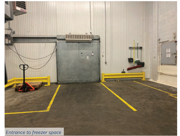
Entrance to freezer space
