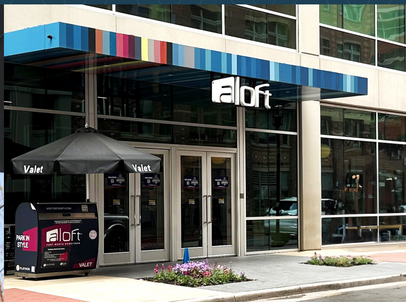
ALOFT HOTEL LOCATED IN ONE CITY PLACE
