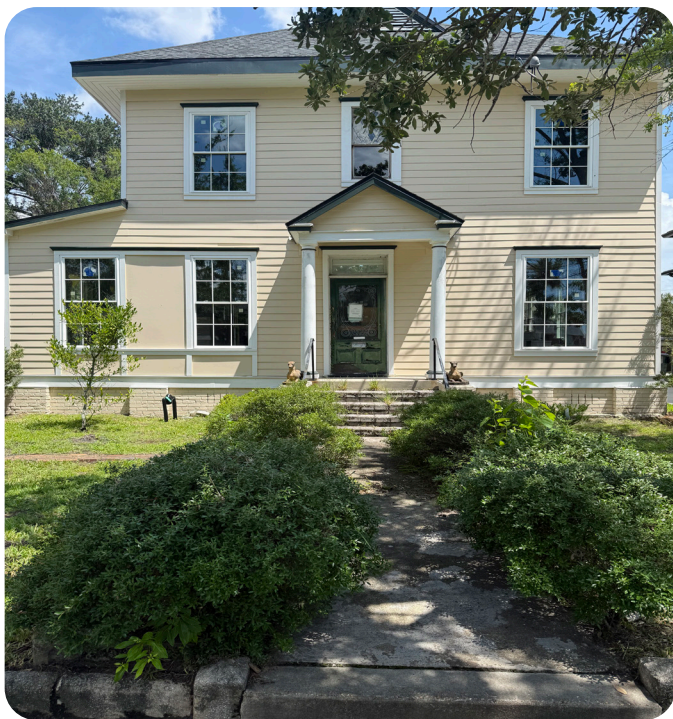
Facing Riverside Avenue, 4290 SF Zoned multi-family residential or commercial
