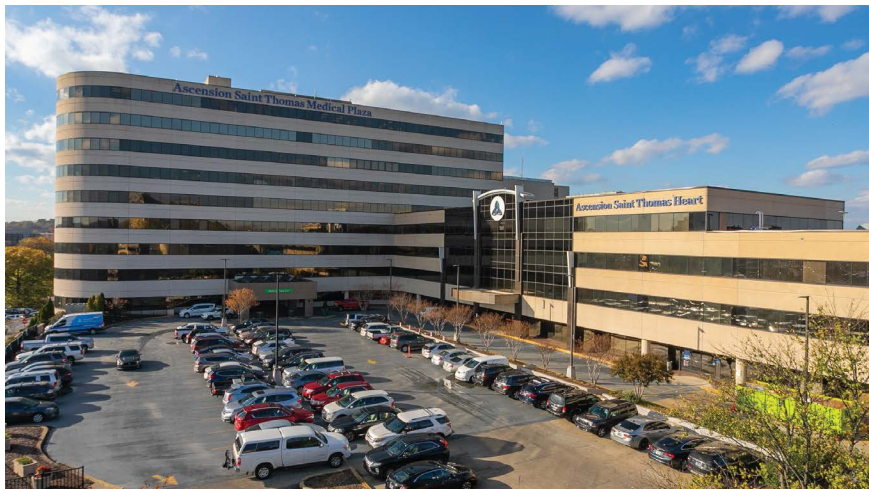
Ascension Saint Thomas Plaza East: 247,228 SF (10 floors) / Heart Institute: 77,105 SF (3 floors)
