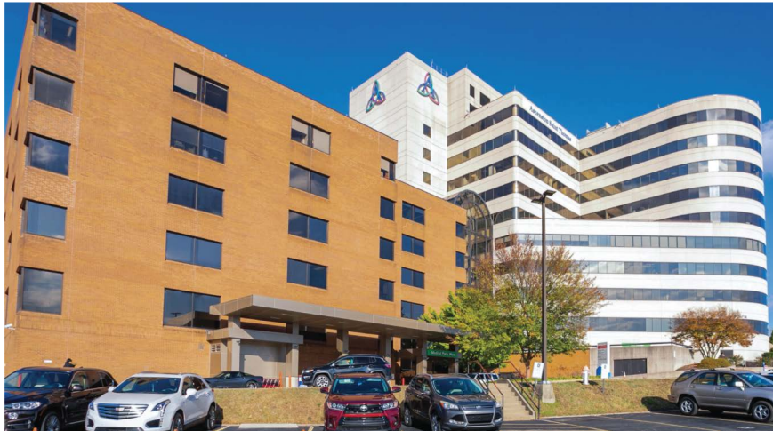
Ascension Saint Thomas Plaza West: 67,085 SF (6 floors)
