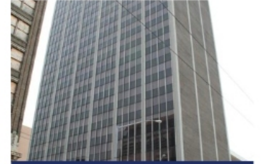
40 W. FOURTH ST. REDEVELOPMENT PROJECT
