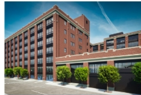
THE DELCO AT WATER STREET 550,000 SF MIXED-USE PROJECT
