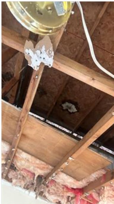
Building 2 interior ceiling
