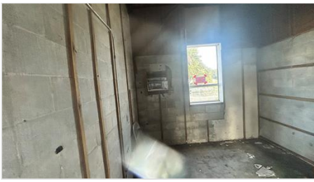
Building 2 interior - kitchen area
