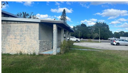
Building 2 - side view from rear
