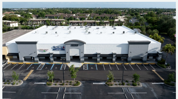
Prominent building identity and multiple storefront entries
