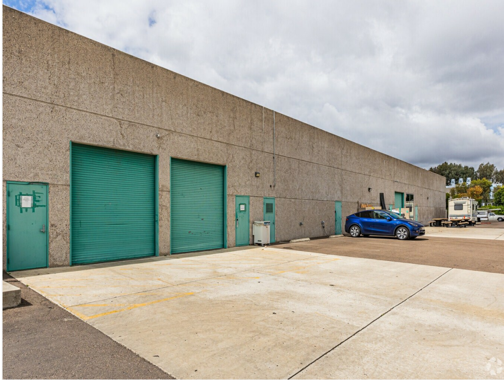
Abundant Shipping Bays
