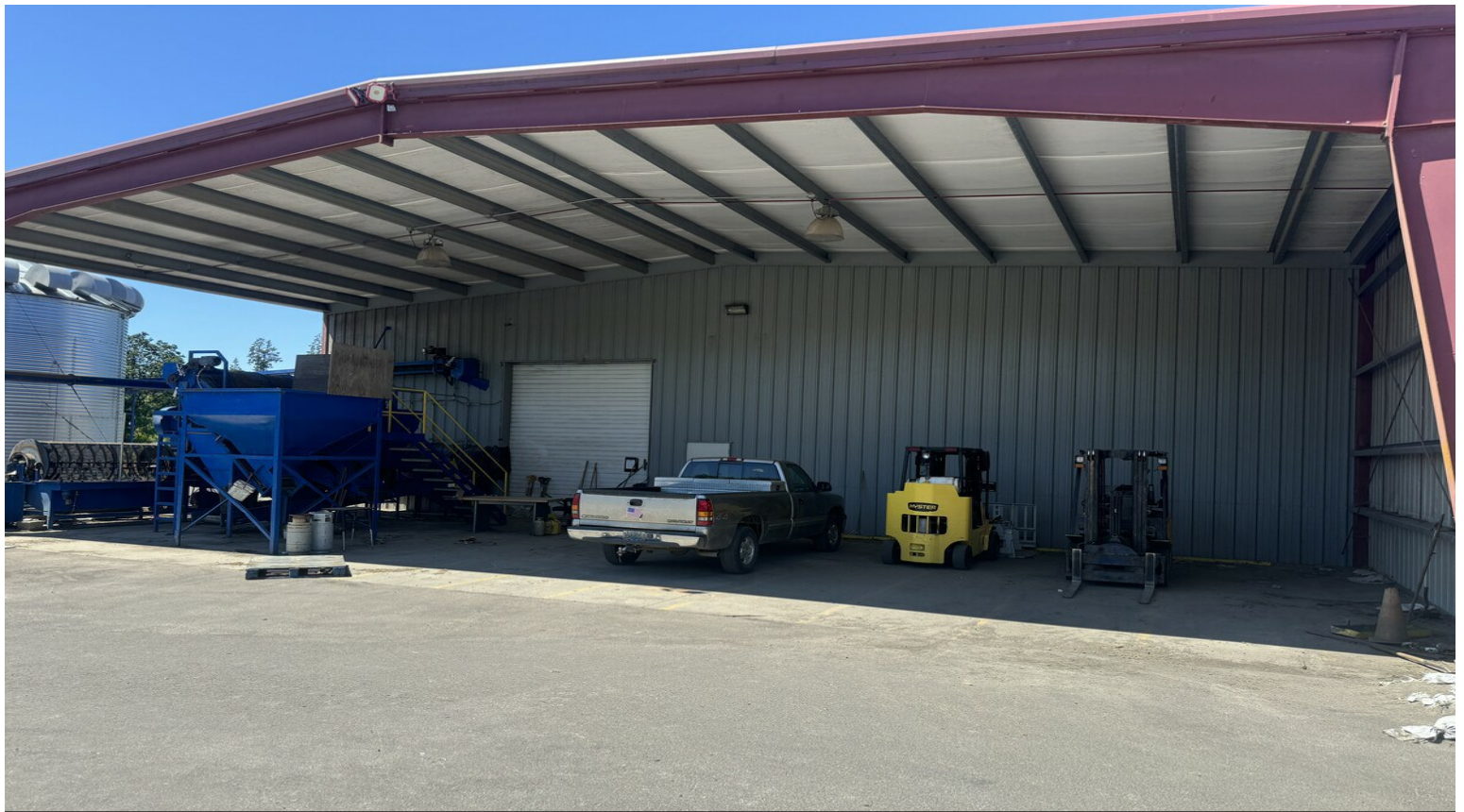
Building 1 - Covered Parking
