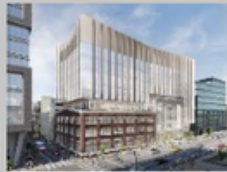
3 2300 Market Street - Under Construction
