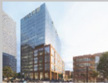
2 2000 Arch Street - Under Construction
