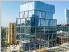
1 2222 Market Street - Completed
