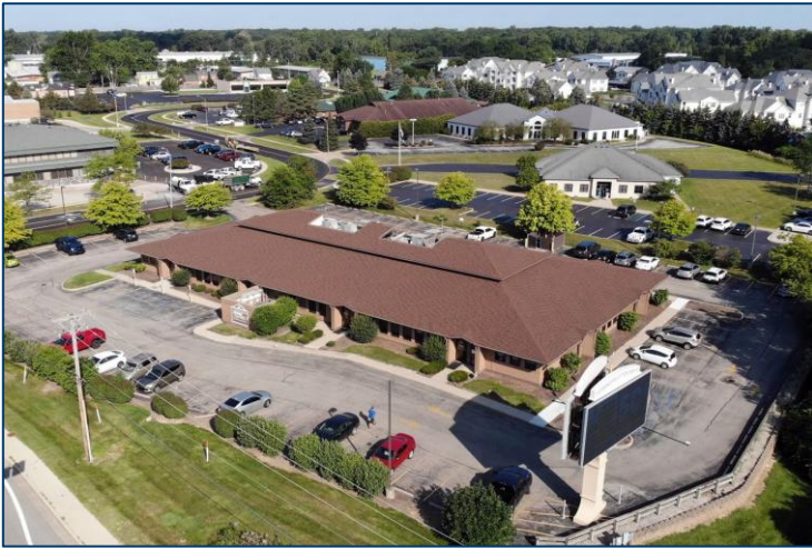
Front of Building – Along Airport Highway
