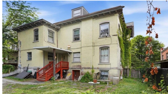
Rear elevation and parking area.
