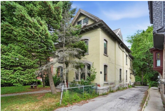
Side elevation and drive.
