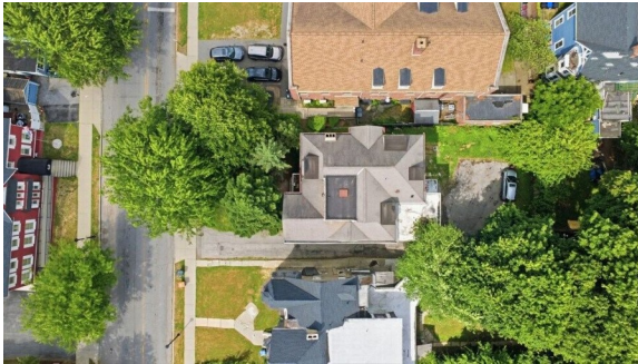
Aerial view. The lot runs deep, with parking behind the building.
