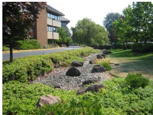
Figure 5.1 Example of vegetated bioswale that catches and filters runoff.
