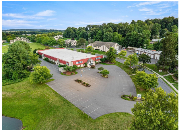
Aerial — Front Elevation
