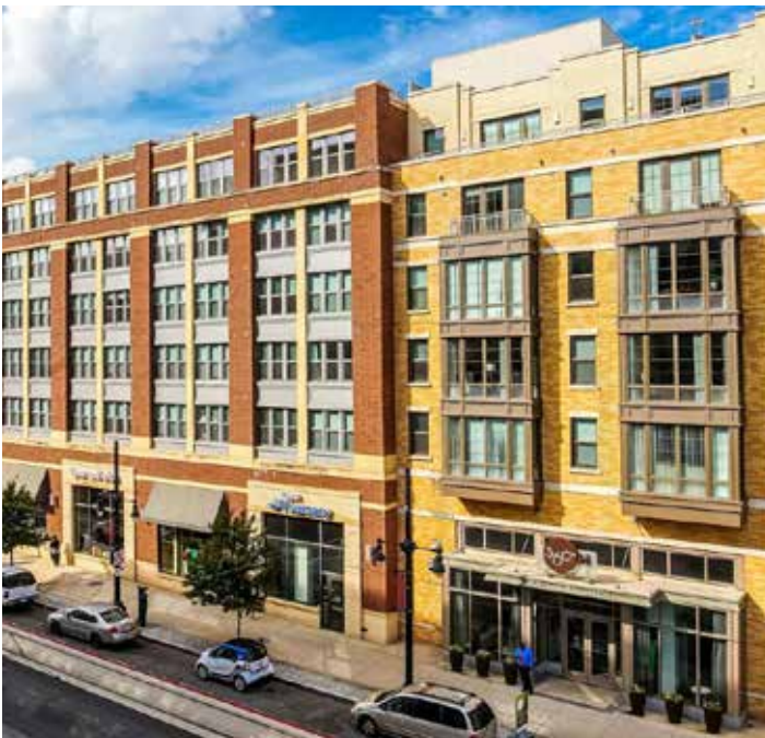
Figure 4.2.11 (b) Appearance of Two Buildings
