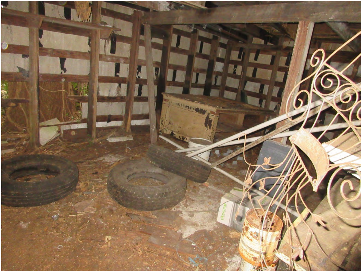
Barn/storage building interior
