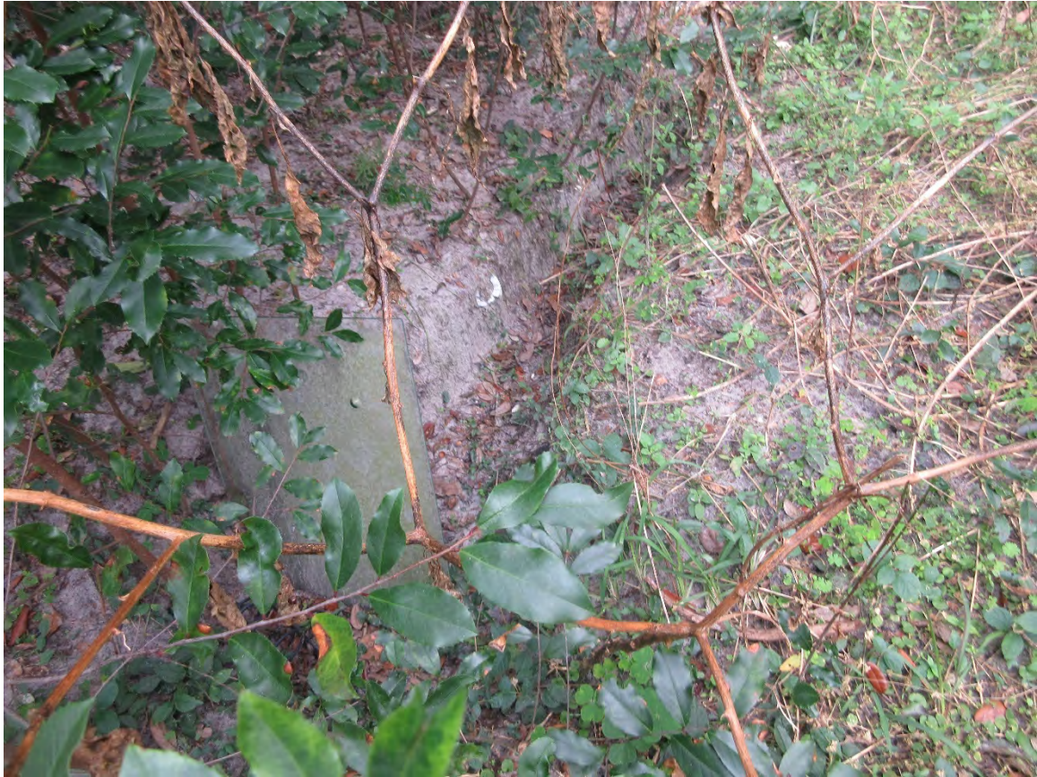
Septic drainage ditch
