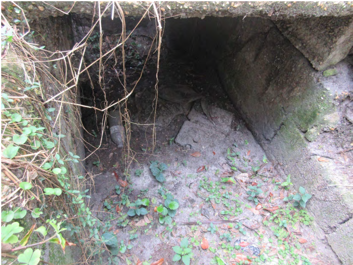
Septic vault (not in use)
