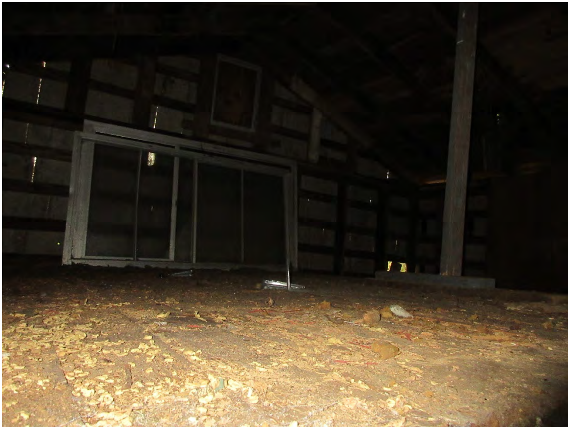
Barn/storage building interior
