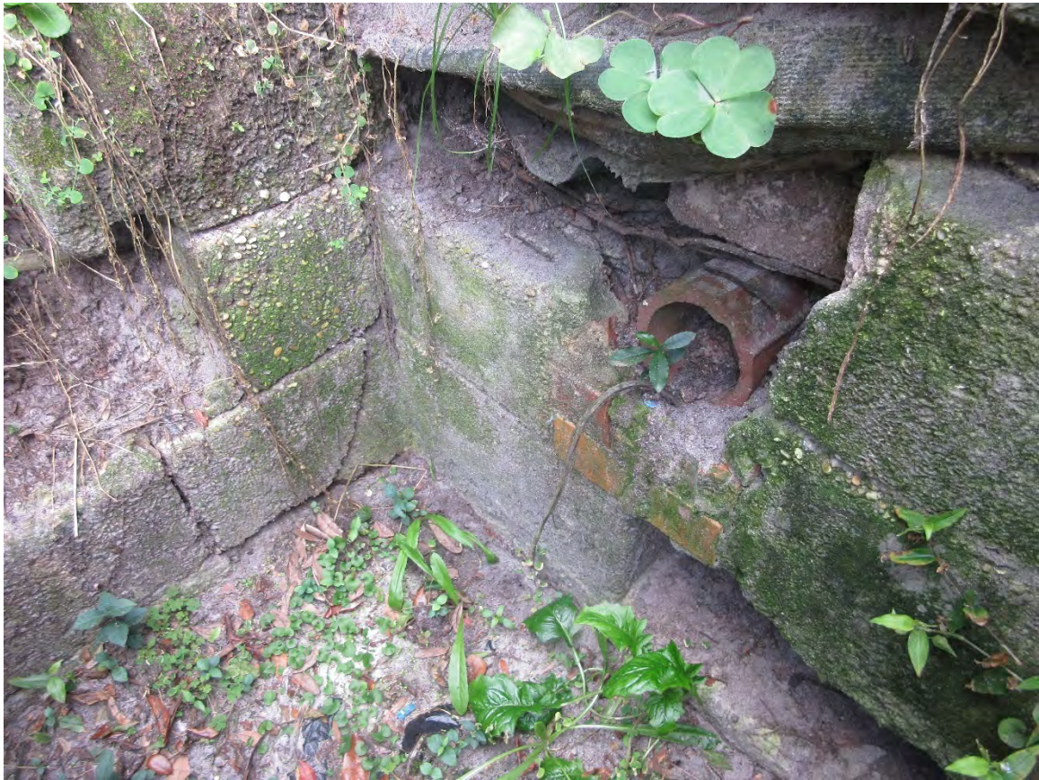
Septic vault (not in use)
