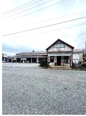
View South Front
