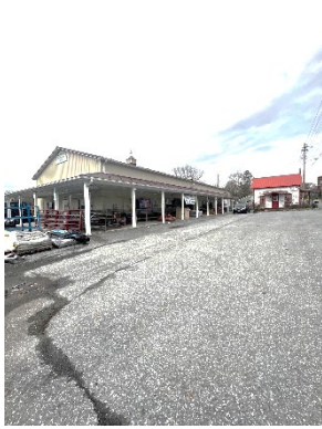
View East Side
