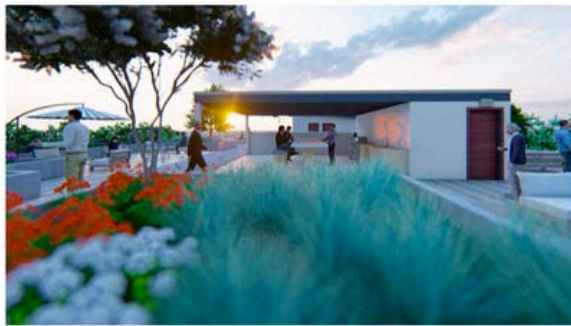
VIEW OF ROOF DECK FROM FROM SOUTH-WEST
