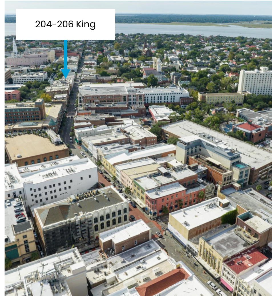
Looking South down King
